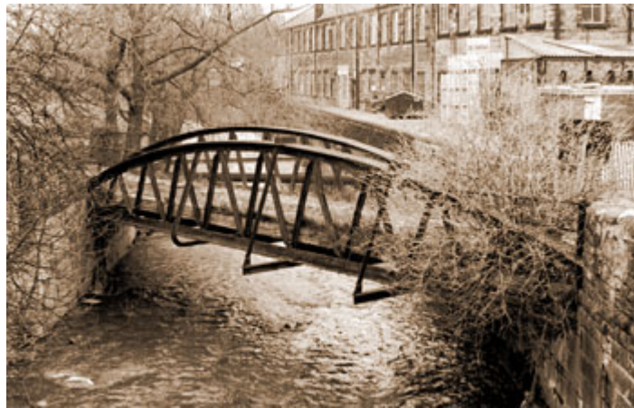
Whaley Bridge Railway.
