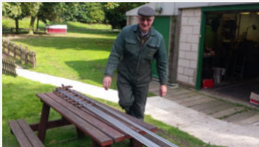
Hon Sec making-up a replacement track section
