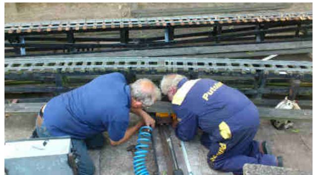
Safety checks being carried out on the south traverser
