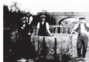
Workers at Funtley brick works
