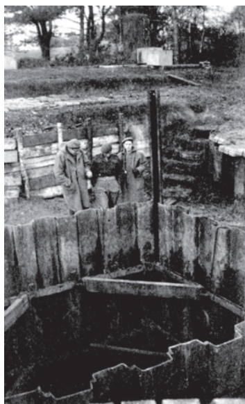
Shuttering in place
