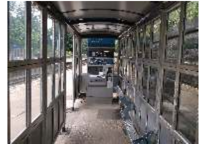
Ticket machine inside the new shelter.
