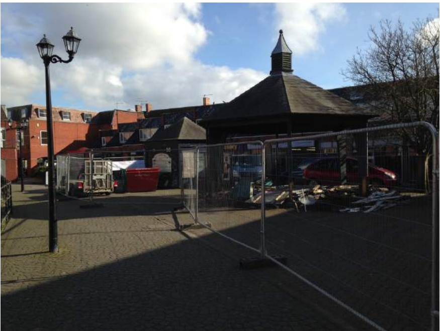
Bandstand being demolished, Riverside Precinct, 17 February 2017.
