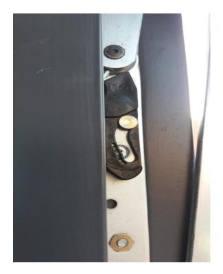
When you close the window you need to release the prop by pushing it down.
