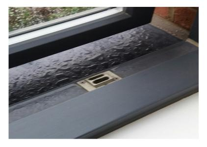
**Fully closed:** pull the window completely shut (using the nearest setting to the windowsill) and turn the handle to the right.
