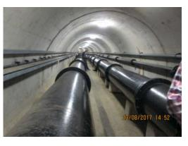
works. Both pipes are just under one metre in diameter and the tunnel is about 80m long.
