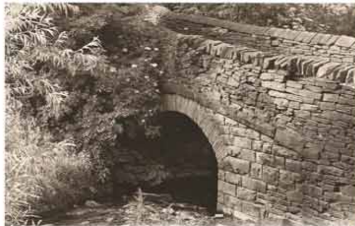
The former pack-horse bridge near Lower Putting Mill
