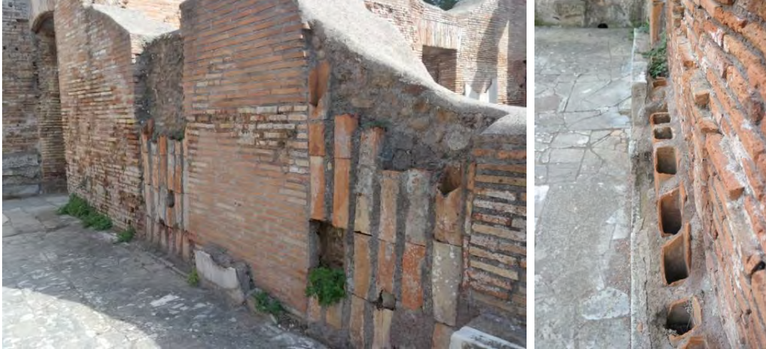
Plate 4 Box flue tiles lining the walls of the forum baths at Ostia, Italy.
