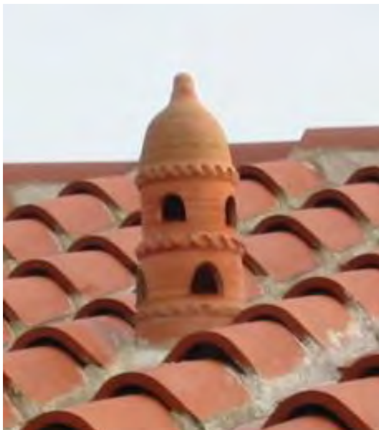
Plate 3 A chimney on a reconstructed Roman roof at South Shields, South Tyneside.
