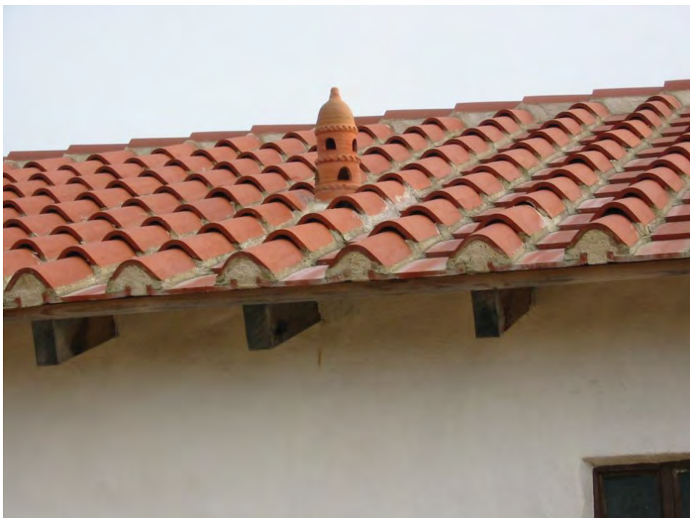
Plate 6 A reconstructed Roman roof of imbrices and tegulae at South Shields, South Tyneside.
