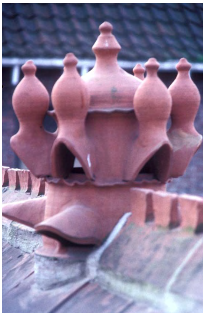
Plate 23 A replica medieval louver on the roof of Barley Hall, York.
