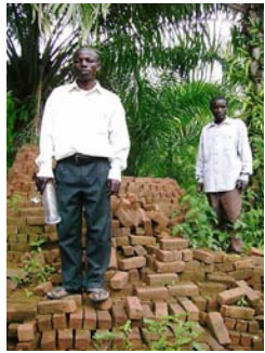
Etando Mukoko Wa Mwabi astride a pile of bricks, fabricated by the local community for the construction of the Trauma Clinic
