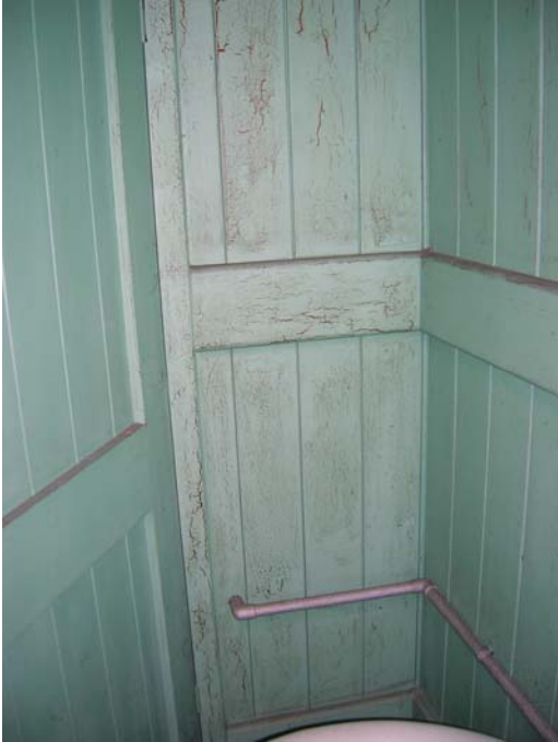
Photograph 9 – Before Conservation Cracking and wrinkling paint on wooden portions of cubicle 3
