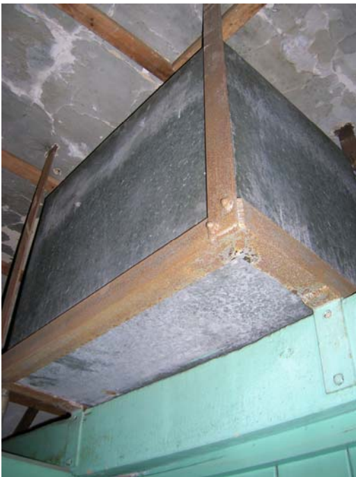
Photograph 47 – Before Conservation Rusting supports to water tank
