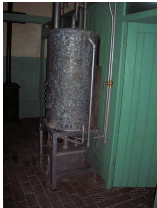
Photograph 32 – After Conservation Boiler and pipes
