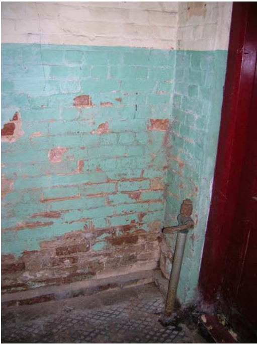
Photograph 17 – Before Conservation Decaying brick in south wall, note missing gas pipes and gas meter
