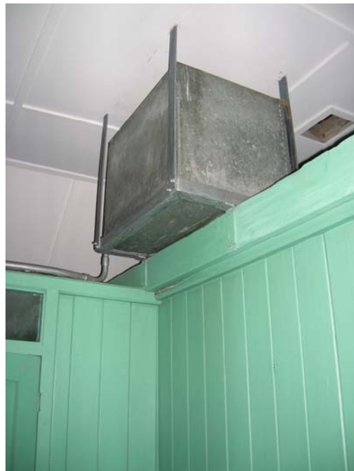
Photograph 48 – After Conservation Water tank seen from inside cubicle 2
