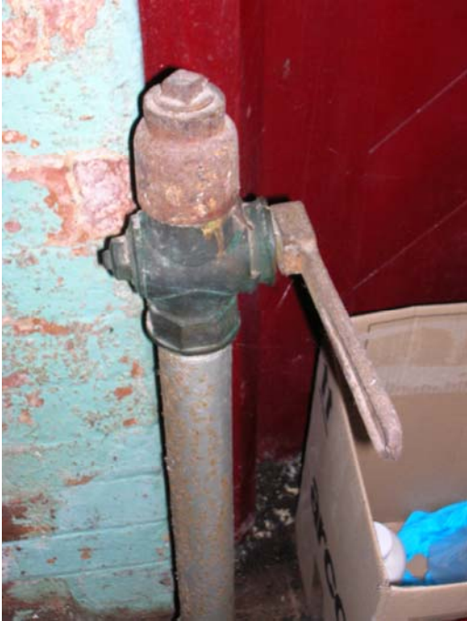
Photograph 37 – Before Conservation Rusting and missing gas pipes
