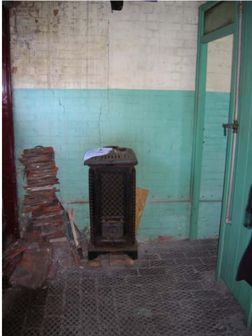
Photograph 1 – Before Conservation View of north wall and rusting stove with missing fluepipe
