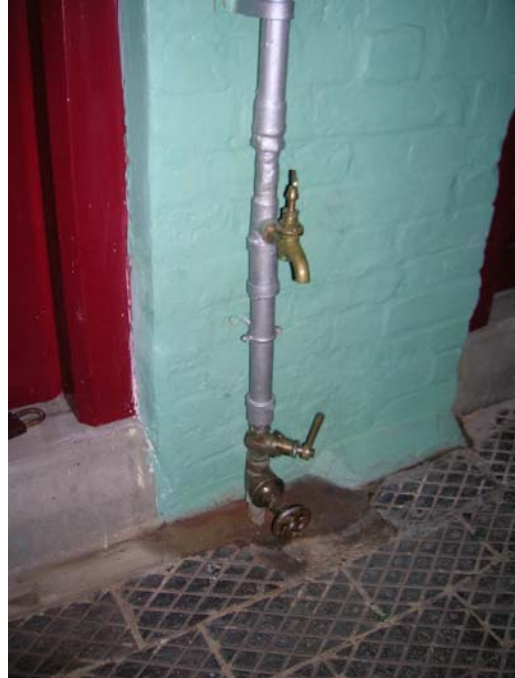
Photograph 20 – After conservation Renewed water pipe
