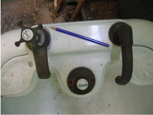
Photograph 33 – Before Conservation Tarnished brass taps
