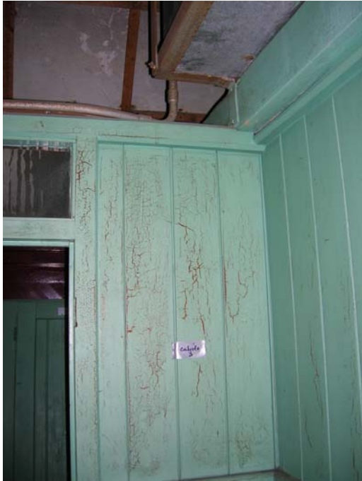
Photograph 49 – Before Conservation General views of cracked paint on partition wall of cubicle 3
