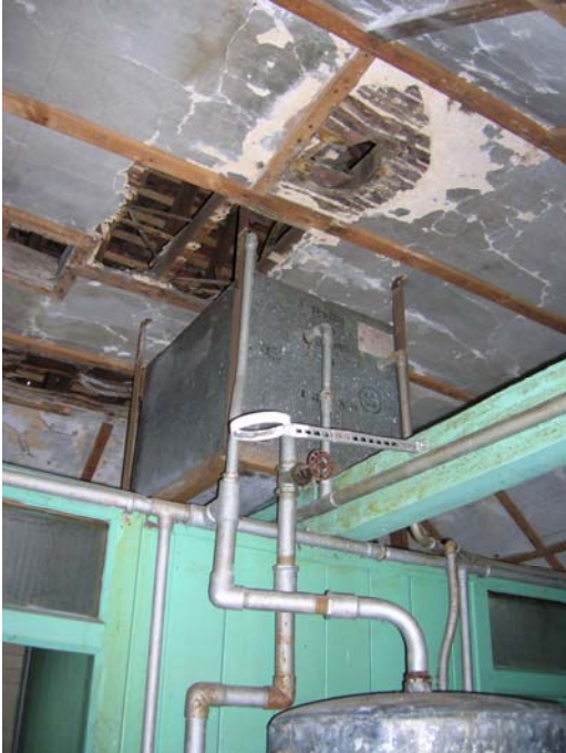
Photograph 45 – Before Conservation Rusting supports to water tank
