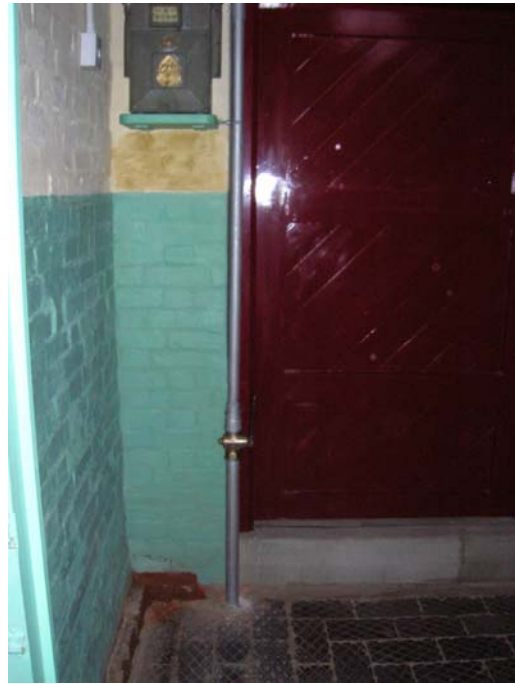
Photograph 18 – After conservation Gas meter with pipes and shelf
