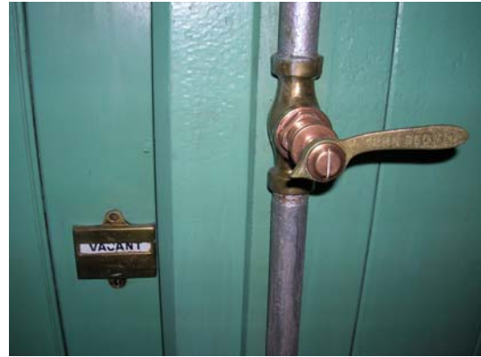
Photograph 30 – After Conservation Water stop valve and engaged sign
