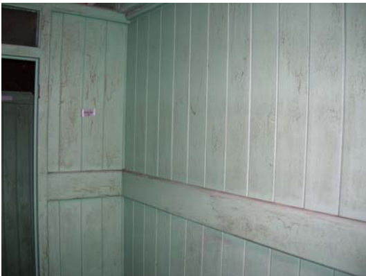
Photograph 43 – Before Conservation Dirt and cracked paint on partition walls of cubicle 3
