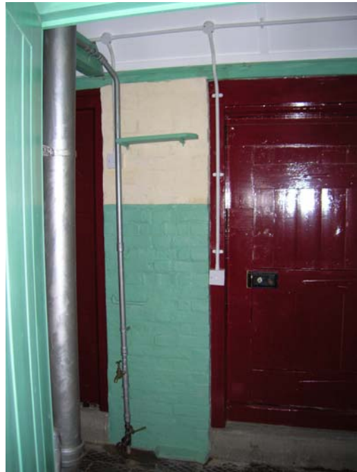
Photograph 36 – After Conservation replaced water pipes
