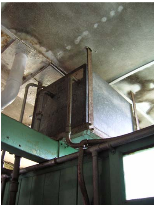
Photograph 27 – Before Conservation Rust water tank supports
