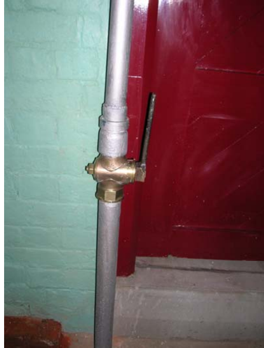
Photograph 38 – After Conservation Replacement gas pipe
