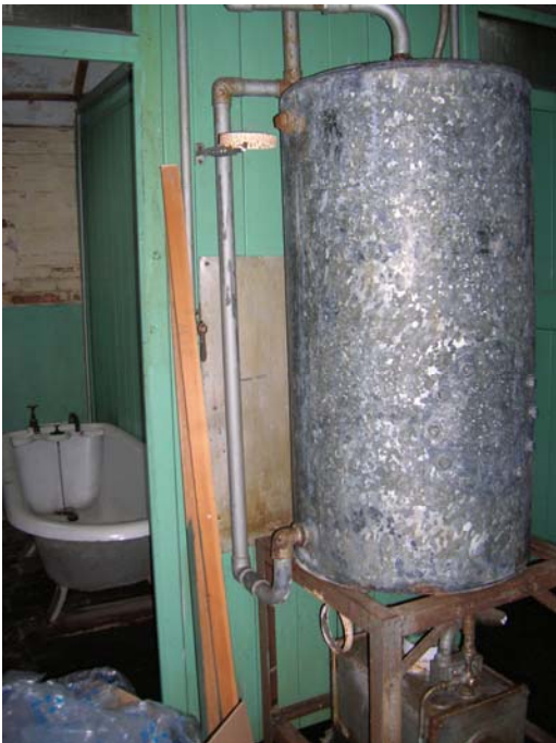
Photograph 39 – Before Conservation Rusty boiler and missing flue pipe outside cubicle 2
