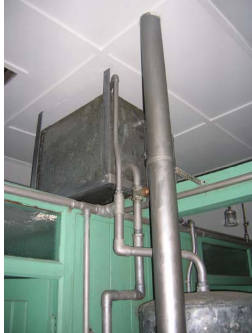
Photograph 46 – After Conservation Boiler flue pipe replacement
