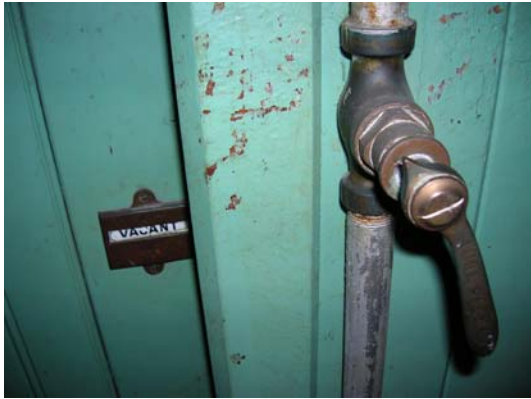
Photograph 29 – Before Conservation Tarnished brass hot water valve and engaged sign on door of cubicle 3
