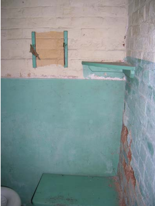
Photograph 15 – Before Conservation Decaying brick walls and missing mirror in cubicle 4
