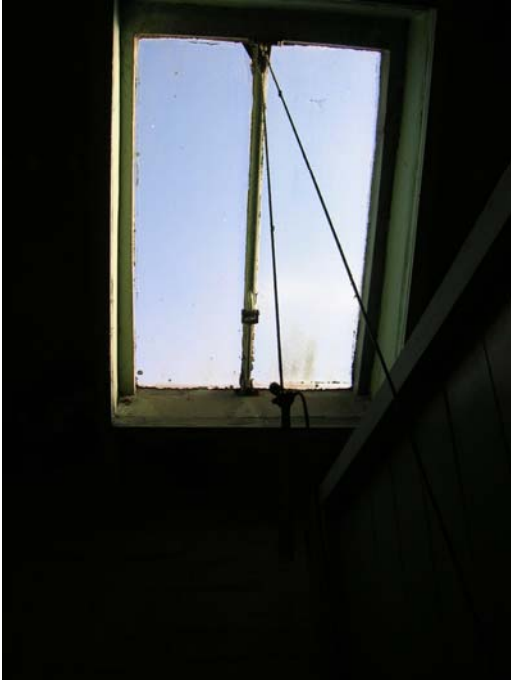
Photograph 13 – Before Conservation Broken window lever in cubicle 3
