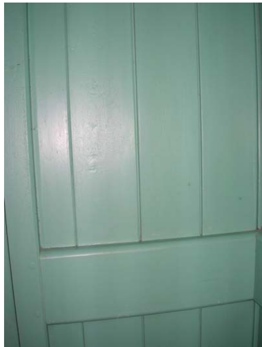
Photograph 12 – After Conservation partition wall, cubicle 3 after cracks and wrinkling had been re-touched.
