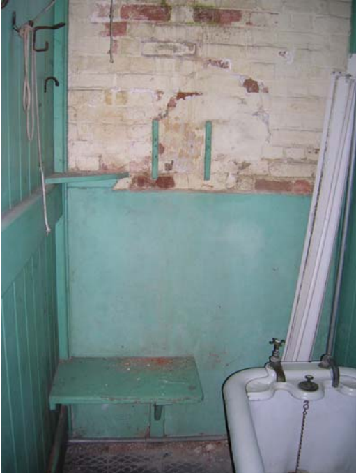
Photograph 7 – Before conservation Cubicle 2, note decaying bricks on wall and missing mirror
