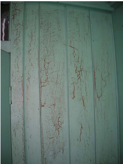
Photograph 11 – Before Conservation Cracking and wrinkling paint on wooden portions of cubicle 3
