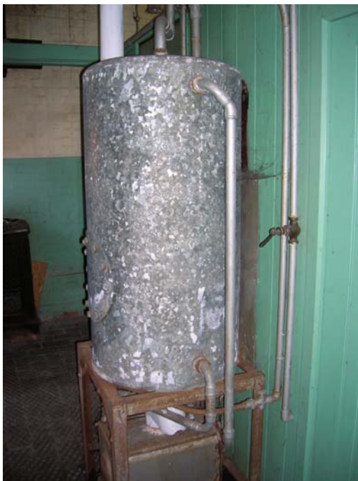
Photograph 31 – Before Conservation Rusting boiler
