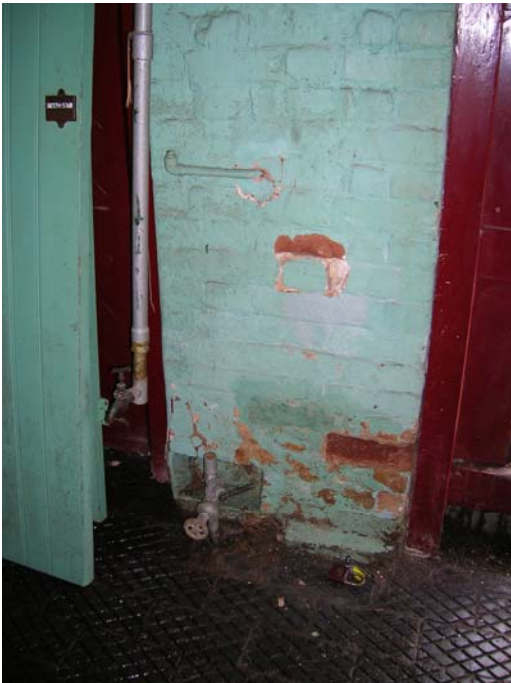
Photograph 35 – Before Conservation Displaced and missing water pipe Against west wall
