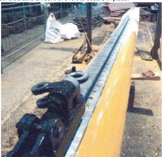
Whilst the new mast was being constructed, the topmast, topgallant, yards and gaff were rubbed down, a few pieces of rotten timber replaced and all were repainted. This work took place alongside the mast construction in No 3 Covered Slip and visitors were able to see all the work taking place at every stage – work was carried out within cordoned-off areas. Outside, the Fighting-top was also given a complete rub down and repaint with some of it's being repaired where rot had taken hold.
