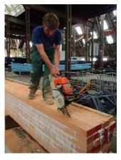
These were then laid and laminated to form a 70 ft long, square sided form which was then cut to shape with a chainsaw and plane (as can be seen in the picture to the left).
