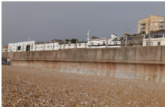
Fig. 13. Curved sea wall, stops waves flooding the pathway.
