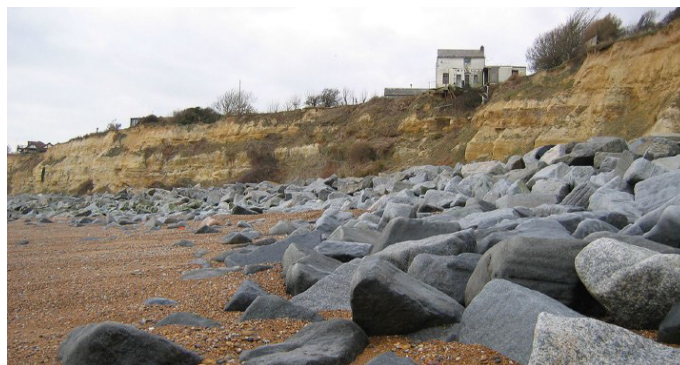
Larvikite revetment protecting the cliffs at Fairlight Cove.
