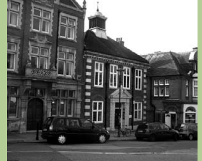
Civic Buildings, 88-94 High Street
