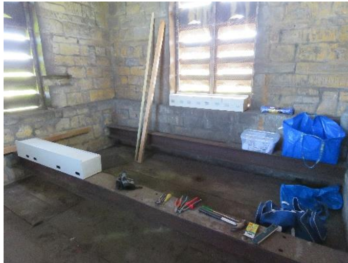
Boxes ready to install
