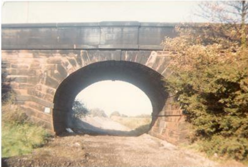
The bridge at Bold as seen looking north in 1983. Photo by Paul Wright
