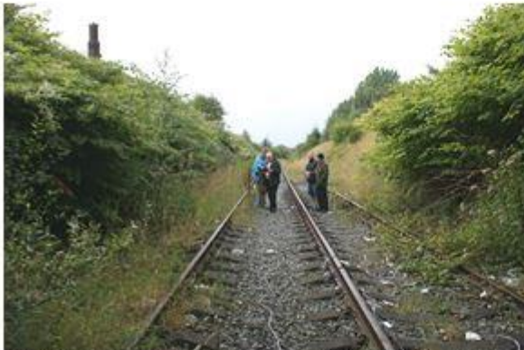
8D Association Members inspect the site of Peasley Cross Station on the 18 th of August 2011.
