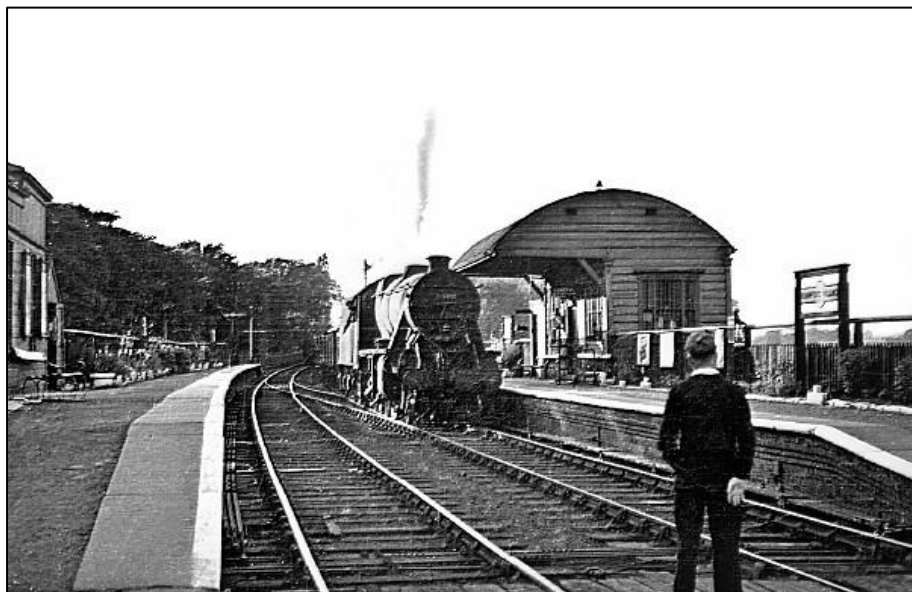
Rainford Village station in 1949. A goods train is seen passing south. It would have just come off the single line section and the signalman is seen waiting to collect the staff. The Healey Mills – Garston train worked by Rod Dixon would have handed over the Randle Junction – Rainford Junction staff in exactly this way. Photo from Stations UK
