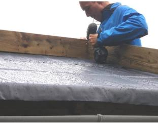
7. Fix the pond liner to the sides using a staple gun.
