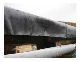
8. Fix a piece of timber along the eave to make a four sided frame.
