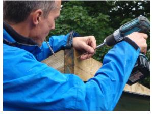
6. Repeat this until you are left with four pieces of wood attached to the apex timber. (The picture below shows 2 pieces attached and this is reflected on the opposite side). Some of the screws will need inserting at an angle.
