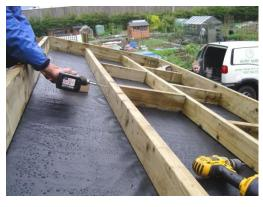
Continue until you are left with several square compartments. Note how the compartments are off set from each other which reduces the pressure (or loading) on the horizontal panels.
