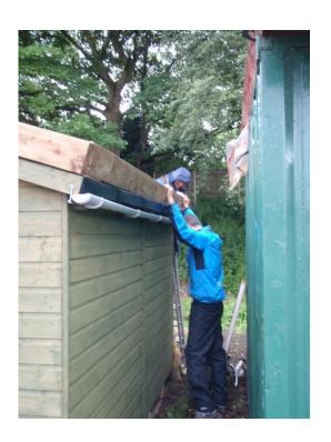
10. To prevent the growing medium and plants from slipping down the roof, a number of wooden panels will now be fixed into the square
