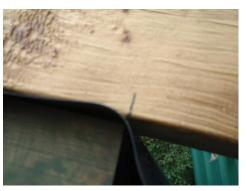
The end of the timber closest to the apex will need cutting at a slight angle to ensure both pieces fit together without any gaps, and it should look like this:
