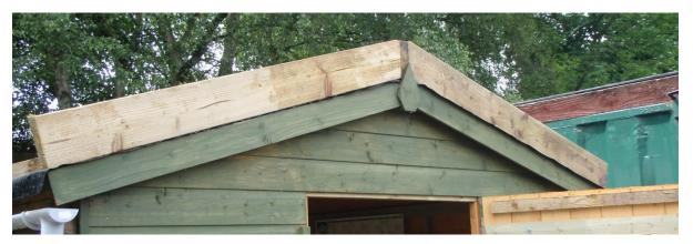
5. Using 5" (13cm) screws, screw through the timber that runs along the apex, into the second piece of wood that has just been measured and cut. Ensure someone is stood at the opposite end to you to hold the apex beam and see it remains in position.
