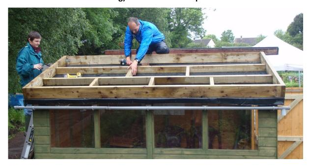
11.Install 90 degree angle brackets in each corner of the inner frame using 2" (5cm) screws
