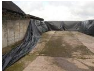
The silage clamp is made of concrete panels which are lined with a new black plastic sheet each year. This photo shows the sheet going up
