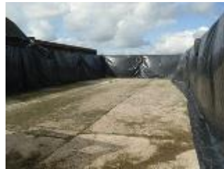
The sheet is up and we're ready for the first load!
