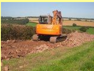
Levelling the stone
