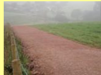
The finished track
