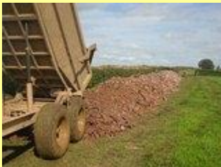
Tipping the stone in place
