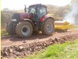
Rolling the stone to compact it
