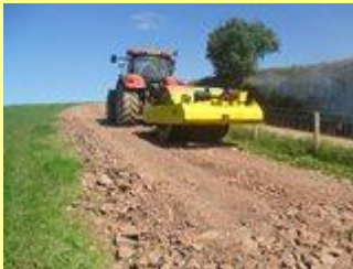
Using the vibrating roller
