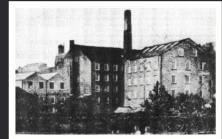
Bottoms mill prior to demolition
