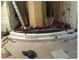
I had hoped we could deal with the level differences and still retain the Victorian tiles in their existing position. To do that, the steps would have to be laid on a slope and that is just not on and I agree with the views of both Wrencon's mason and the architect that the steps must be level. A keen eye would see it was not level and that would never be acceptable.
