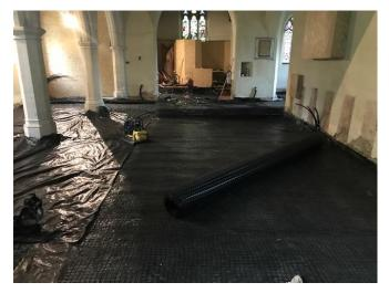
Following on from last week the first picture shows the glass insulating layer being put in place over the geotextile material.
