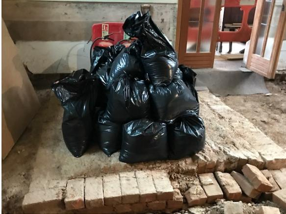
shows this being carried out. The vault roof passed this test so we have a solution with little additional cost. Above part of the vault there will be a cupboard, but the area where there will be an open floor it seems that the depth available above the vault roof will not be sufficient to enable underfloor heating to be installed so there will be a cold spot over this area, which will be compensated for by a radiator against the wall at this point.
