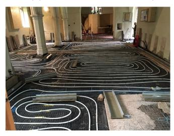
veneered panels so that it doesn't look out of place with the rest of the furniture. The under-floor heating provides background heat and there will be radiators to provide a top-up when needed. I am told the pipework has a life expectancy of at least 400 years!
