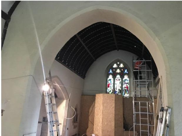
Work has now started on laying the stone floor tiles. There was a bit of a delay while the electricians took over virtually the whole site, working at both high and low level. By the end of the week they had pretty much completed their 'first fix'. The picture shows them putting cables in the Chancel ceiling which was the last part to be completed.
