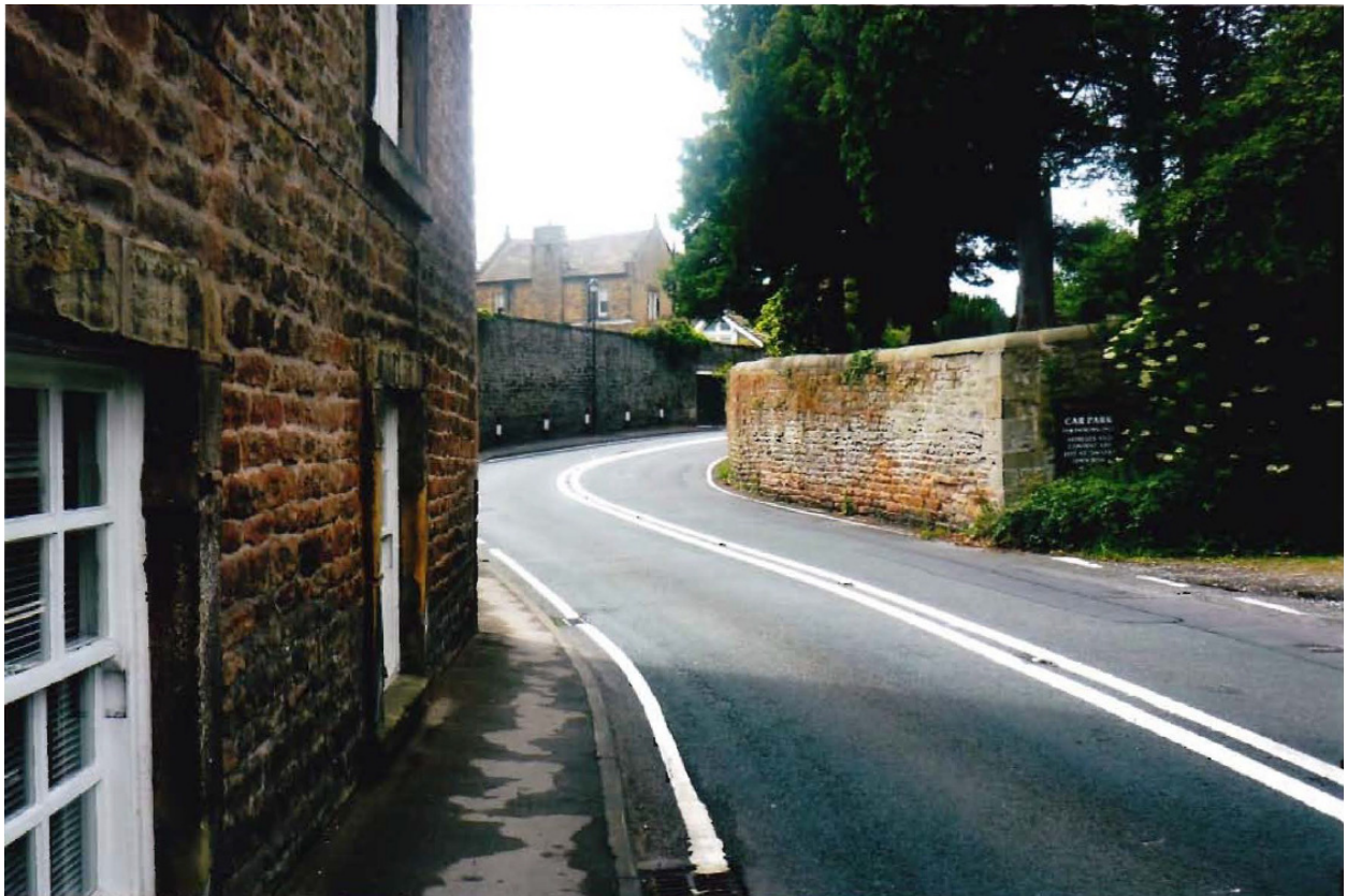
Figure 1 – The geography of Church Brow, illustrating tight blind bends, narrow pavement (68cm width), residential accesses and retaining wall.
