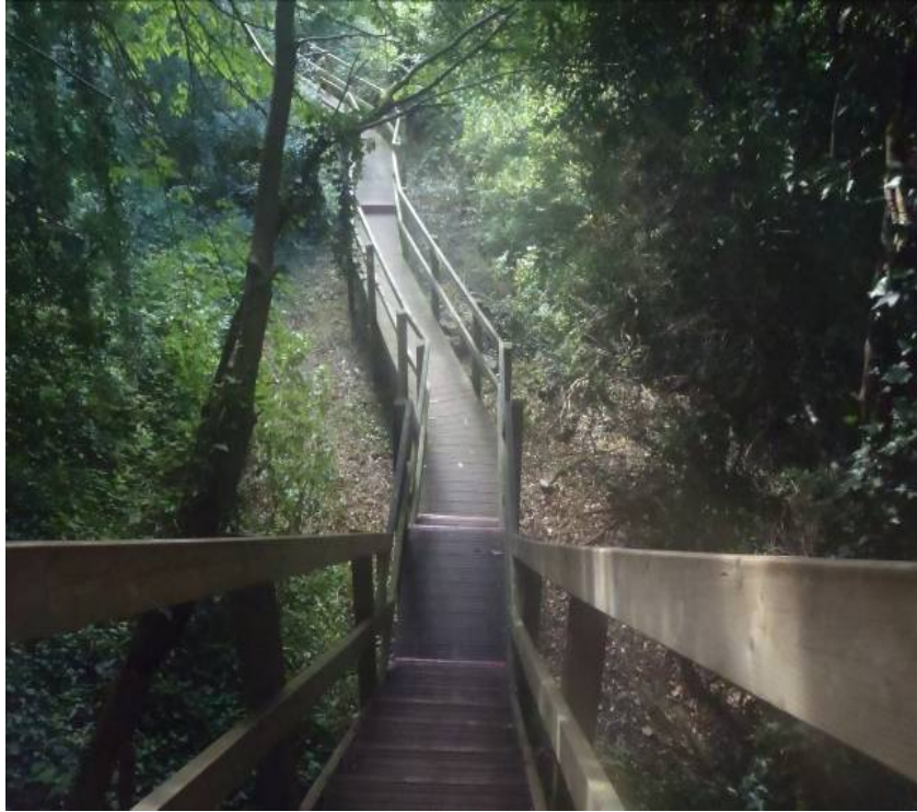
Photograph2: Steps and boardwalks allow access to otherwise inaccessible areas.
