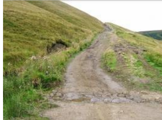
Photo: After DCC repairs
