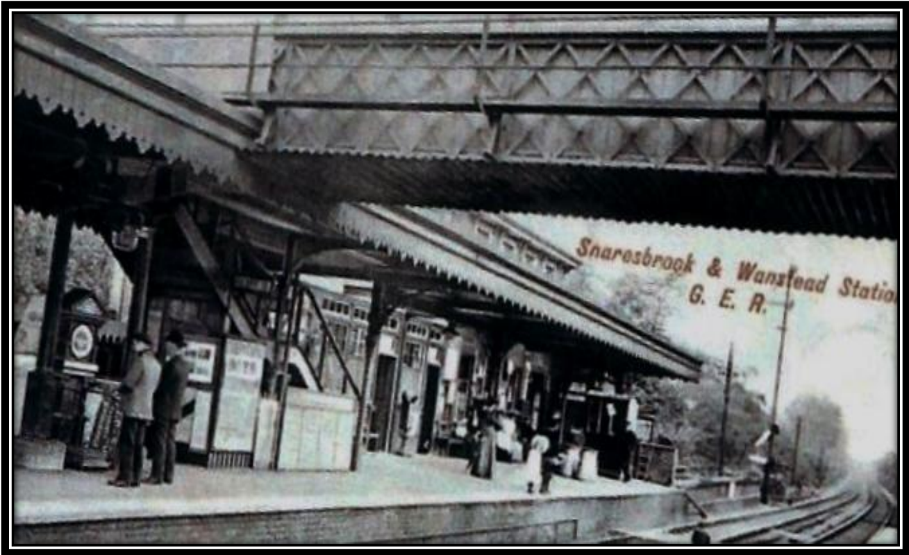
Snaresbrook Station Platform and Bridge
