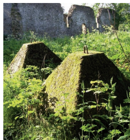
Concrete war defences at Waverley. Phot: June Chatfield
