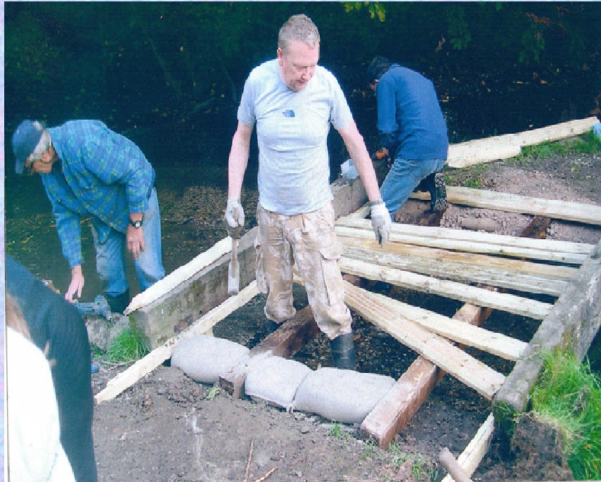
Replacement of the existing bridge Photo: A. Baker
