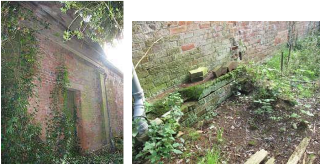
Figure 5: Back elevation of the Orangery showing foundations of former boiler house
