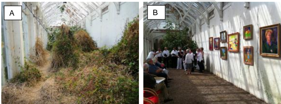
Figure 4: The inside of the Orangery (a) before clear out (b) Open Day in September 2012
