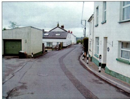
Figure 8 - Middle of the village. This area is particularly hazardous for pedestrians. A marked walkway should be provided as well as arranging for "slow" signs to be painted on to the road. Some of the bollards are damaged and need to be replaced. However, the materials used for these make them very modern in appearance. Perhaps wooden posts with reflective patches would be more suitable and in keeping with the area. A rope or chain could be added between the posts to make a physical barrier between the car and pedestrian. The addition of "SLOW" painted on the road surface, or raised painted strips may be an additional help along this narrow stretch of road.
