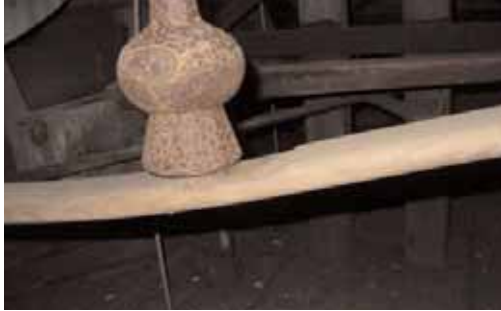
Tenor flight is colliding with slider bar at West Haddon.
