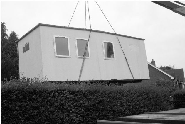
New (second-hand) classroom being installed. Photo by courtesy of Dave Watson
