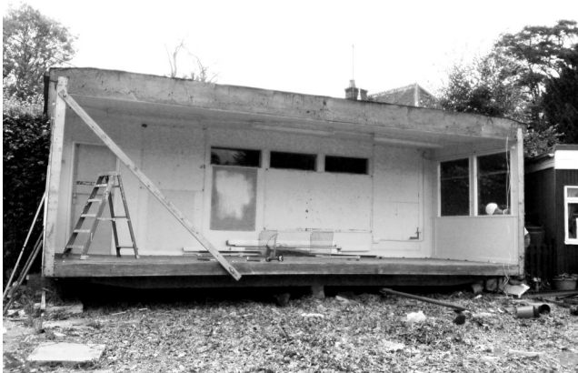
Demolition of old classroom Photo by Jennifer Smith
