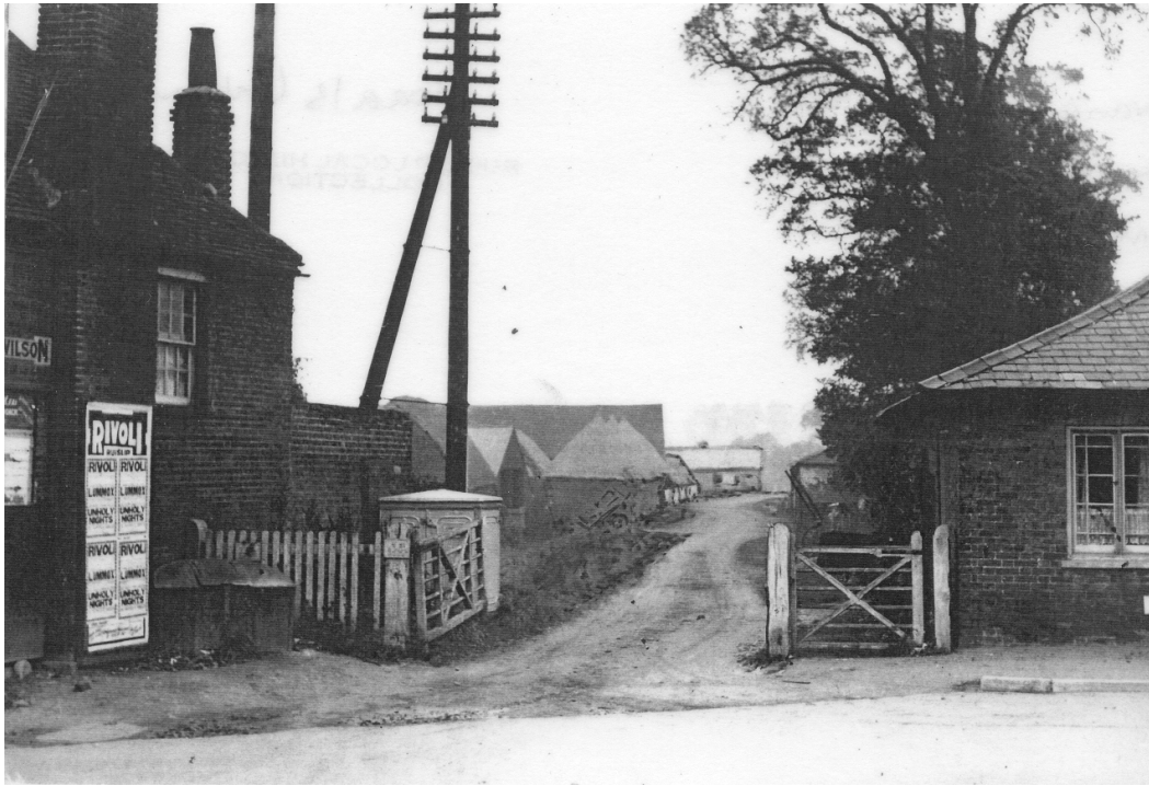
Entrance to Manor Farm c.1930 showing the rickyard, the Little Barn, the old Cow Byre and the stable block in the distance.
