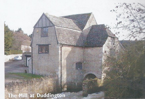
The Mill at Duddington
