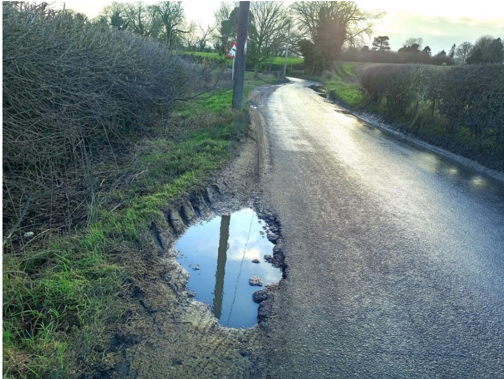
Knaresborough Road, close to Thorpe Farm , from Ripon coming back towards Bishop Monkton. Notice erosion and deformation of roadside. Is this post legally sited, so close to the carriageway?
