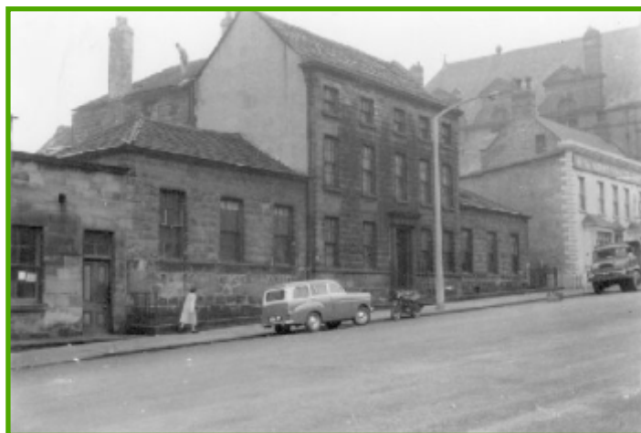
Micklegate House, 1950's - now demolished Horsefair (note Horsefair Vaults to the right)
