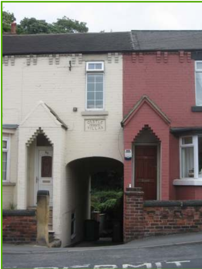
Detailing on North Baileygate
