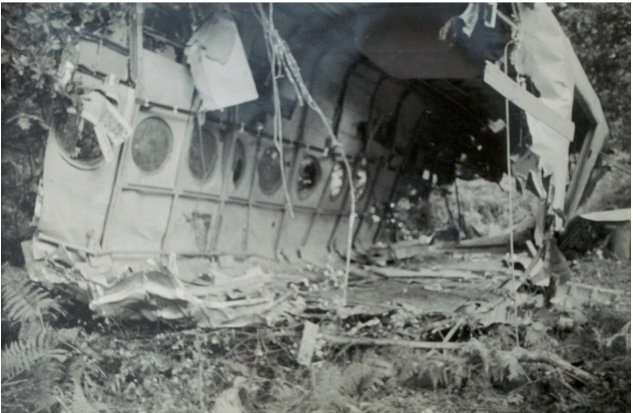
Fig. 3 - York. Fuselage showing damage to starboard side
